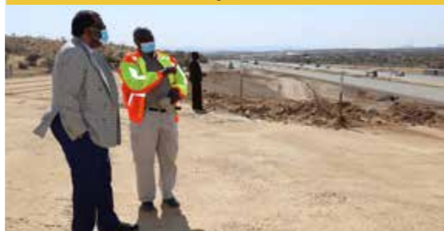
H.E. President Geingob inspecting the WHK-Hosea Kutako Road
